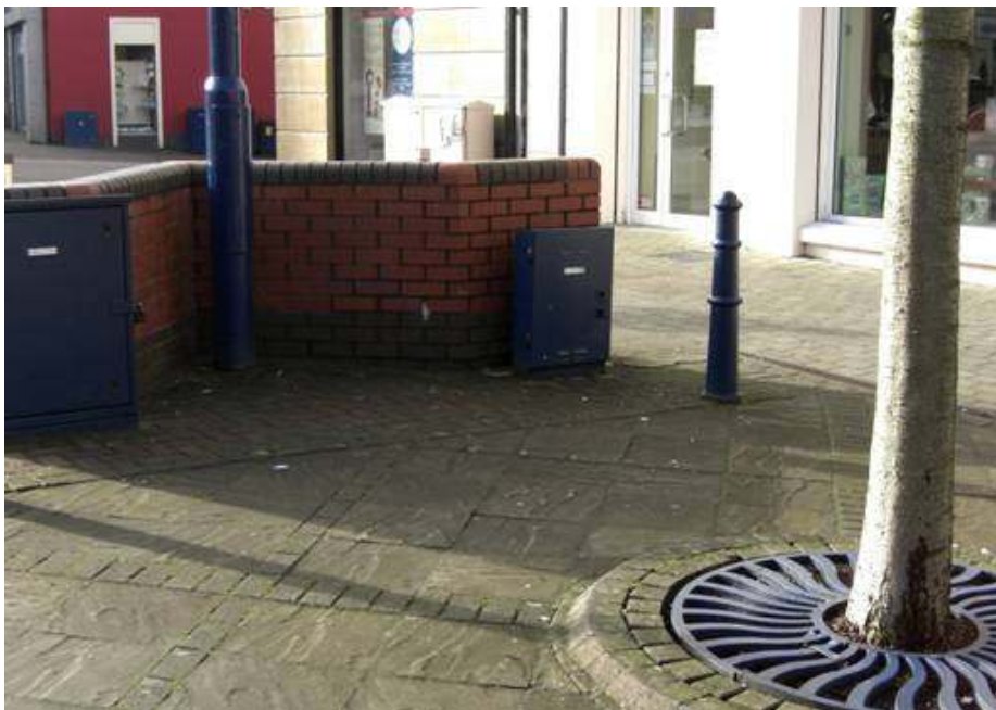
Utility boxes, street lighting, bollards and tree guards painted in same colour (despite different agency ownership)
